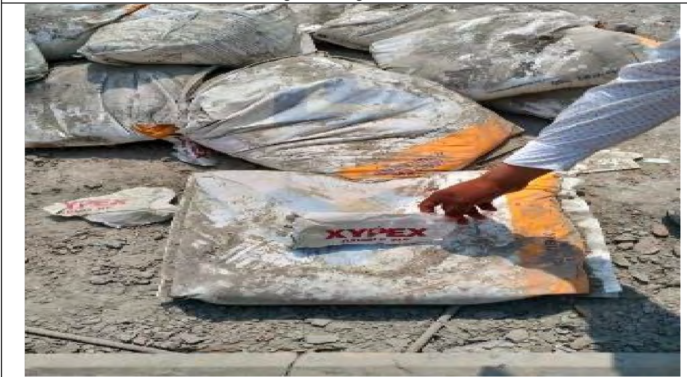
Additive (Xypex) used with SRC to provide water -proofing
