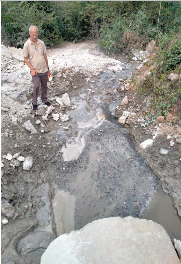
Slurry deposited from Sedimentation tank has choked the nala due to cementing. This needs to be cleared on regular basis.
