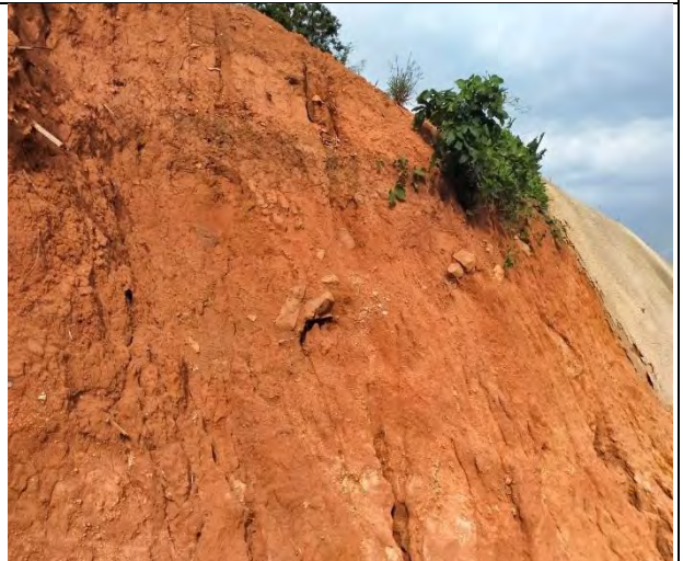
Side slope issues requiring action for protection including measures like Bio-engineering
