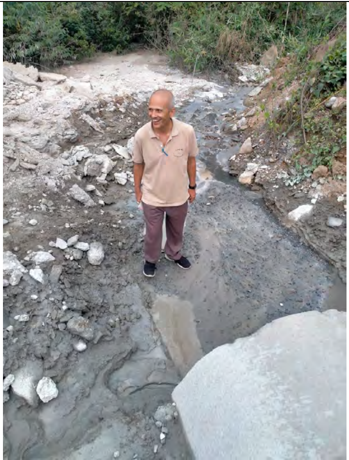
Slurry deposited from Sedimentation tank has choked the nala due to cementing. This needs to be cleared on regular basis.
