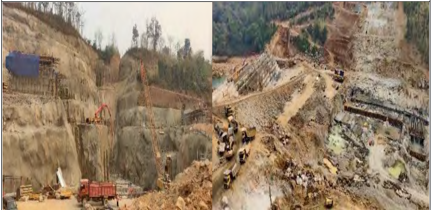
Construction Activities at Powerhouse and Dam Site
